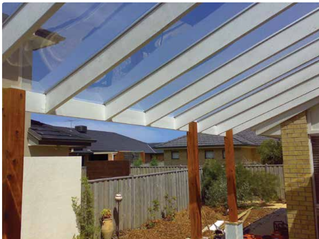
Project: Private home, Point Cook, Australia | Application: Pergola | SUNGLAZE™ Type: Clear 3mm
