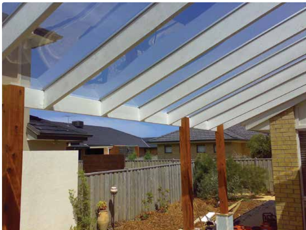
Project: Private home, Point Cook, Australia | Application: Pergola | SUNGLAZE™ Type: Clear 4mm
