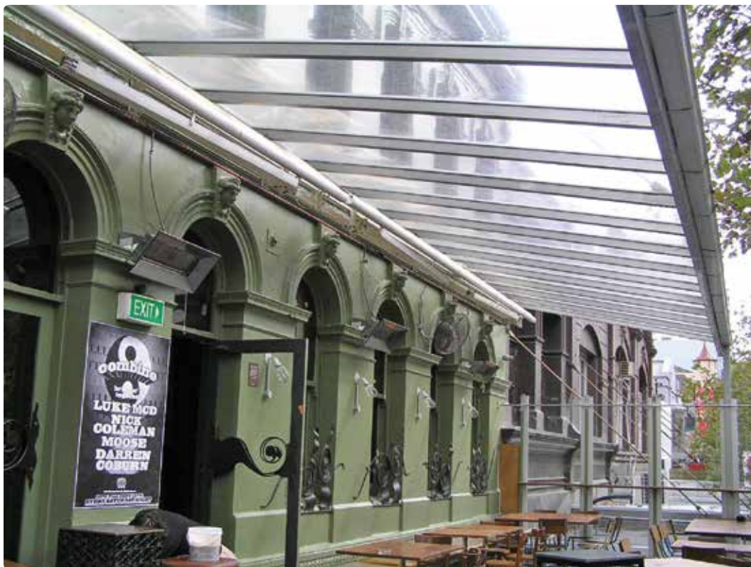
Project: The Lounge Bar, Melbourne, Australia | Application: Canopy | SUNGLAZE™ Type: Clear 3mm
